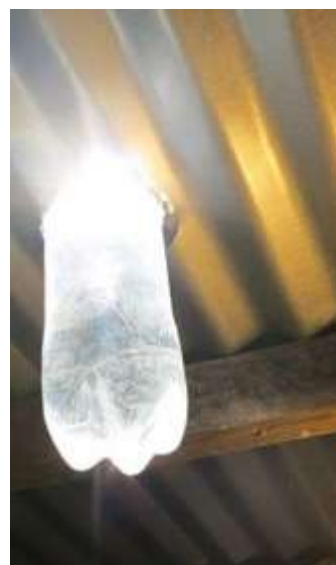
Figure 15: A litre of light embedded in shack roof
